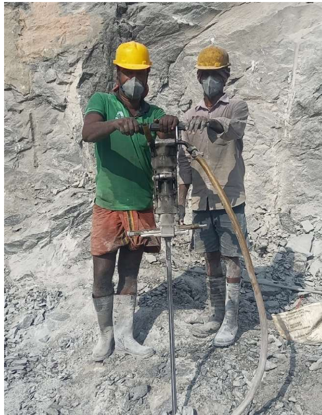
Fig 6: Drilling of blast holes using jack hammer
