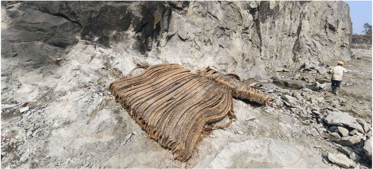
Fig 13: Muffling arrangements to control the Fly rocks
