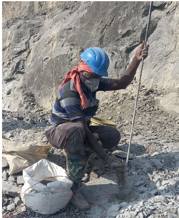
Fig 11: Stemming of Blast holes
