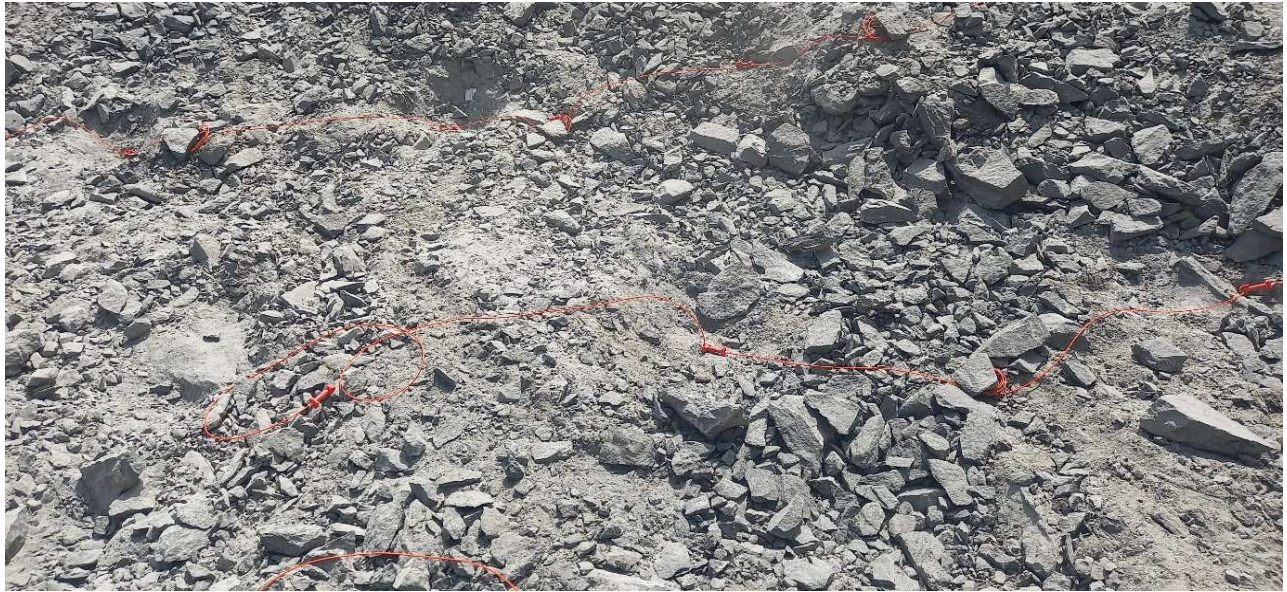
Fig 12: Charged Holes
