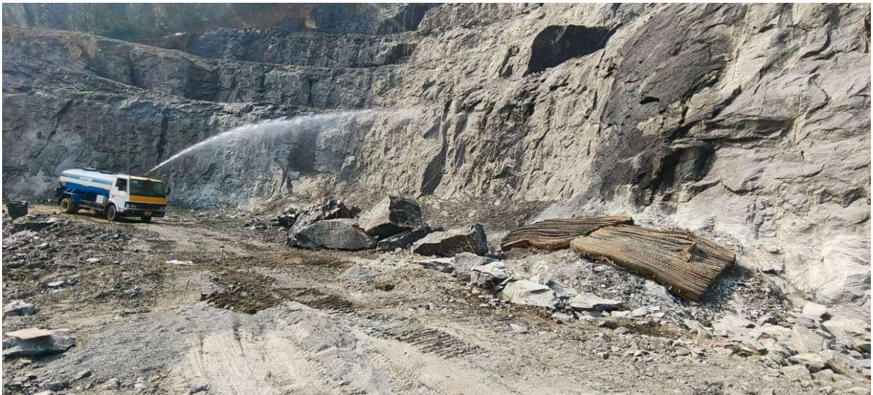
Fig 14: Water spray system and water sprinkled face
