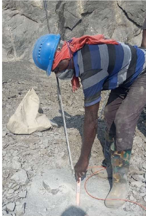
Fig 10: Charging of Blast holes
