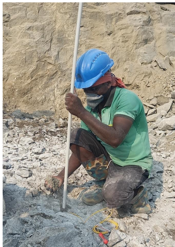
Fig 10: Stemming of Blast holes
