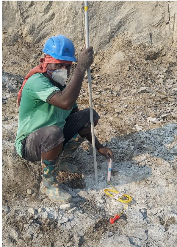
Fig 9: Charging of Blast holes
