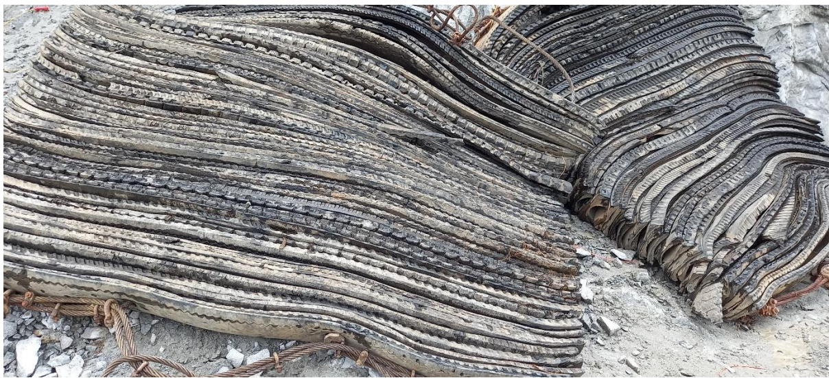
Fig 12: Muffling arrangements to control the Fly rocks
