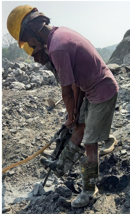
Fig 6: Drilling of Blast Holes using Jack Hammer
