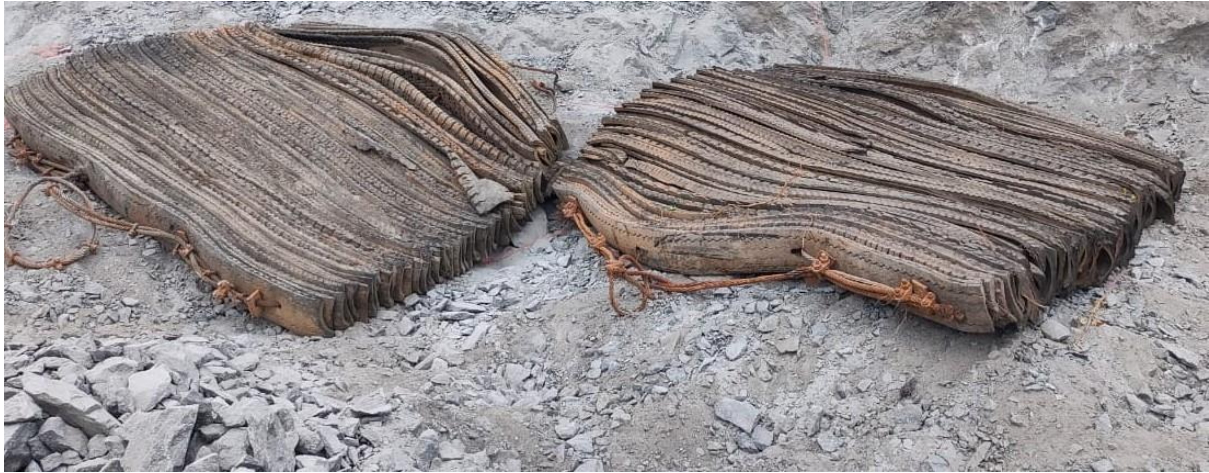
Fig 13: Muffling arrangements to control the Fly rocks
