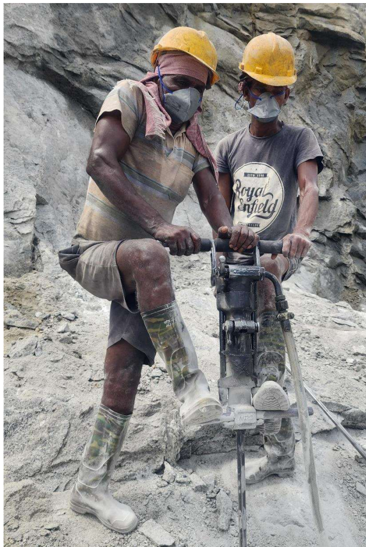
Fig 6: Drilling of Blast Holes using Jack Hammer
