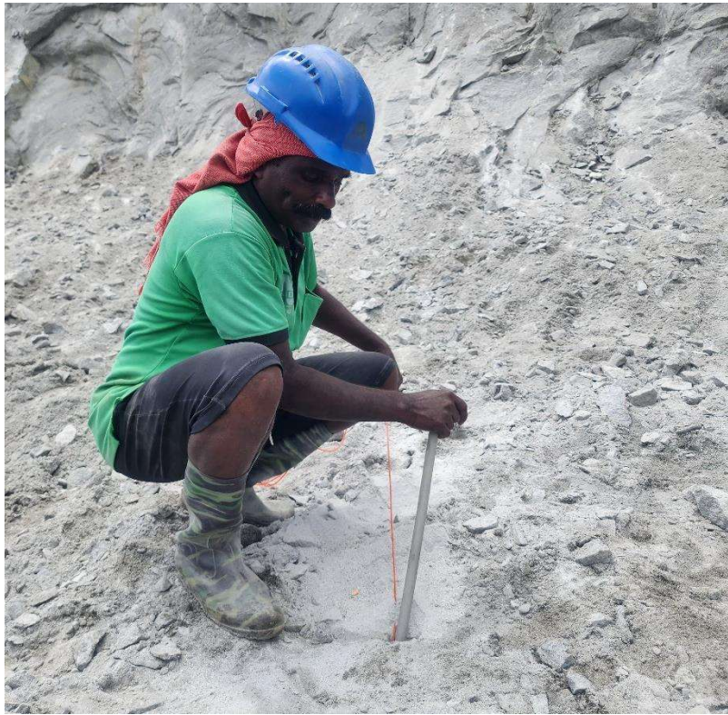
Fig 10: Stemming of Blast holes
