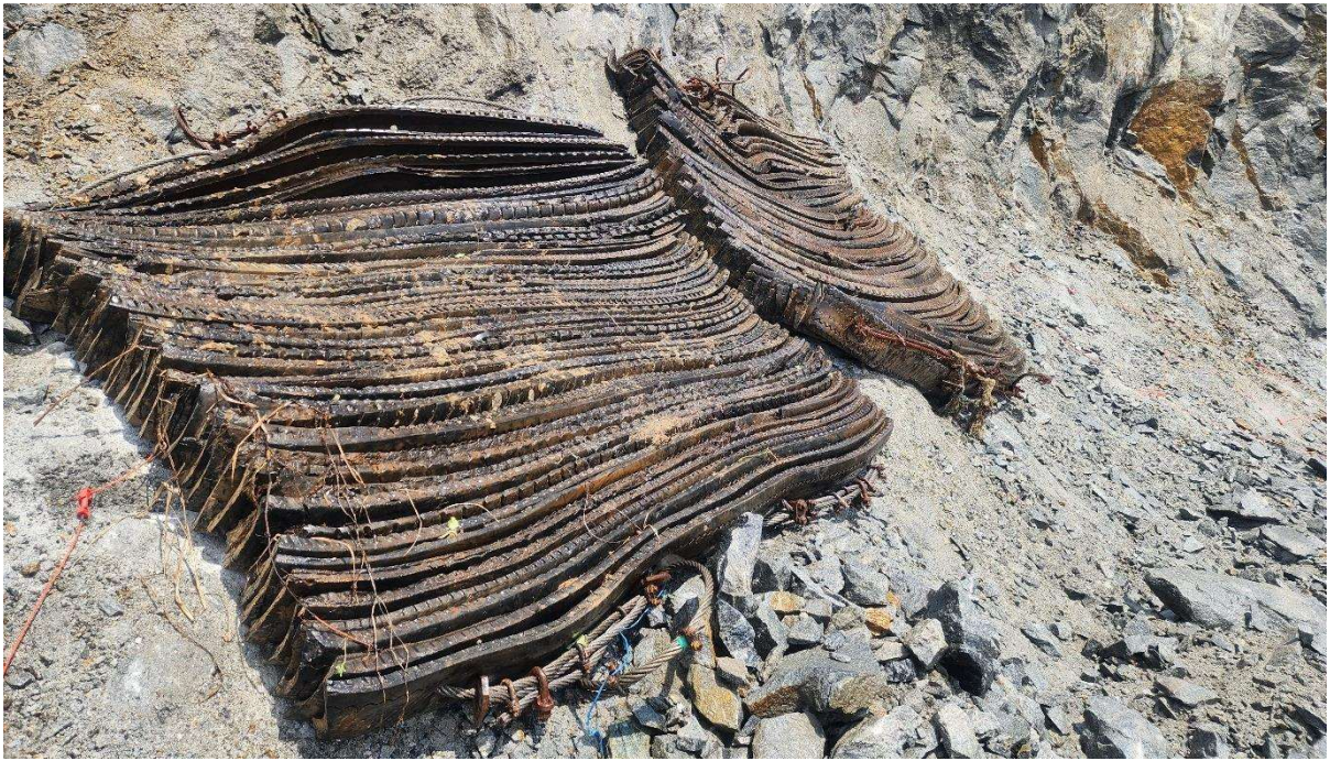
Fig 12: Muffling arrangements to control the Fly rocks
